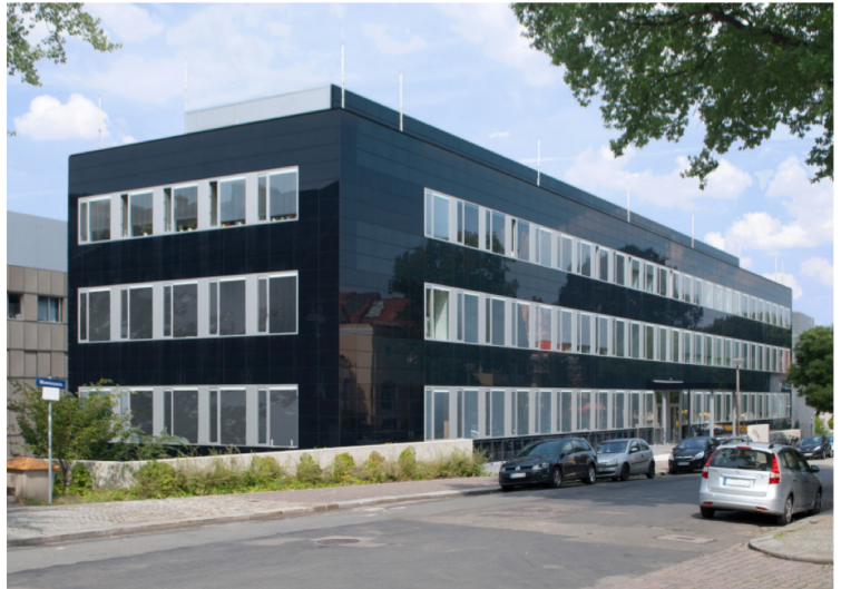
CIGS building-integrated facade with CIGS modules by (image: Manz AG)
