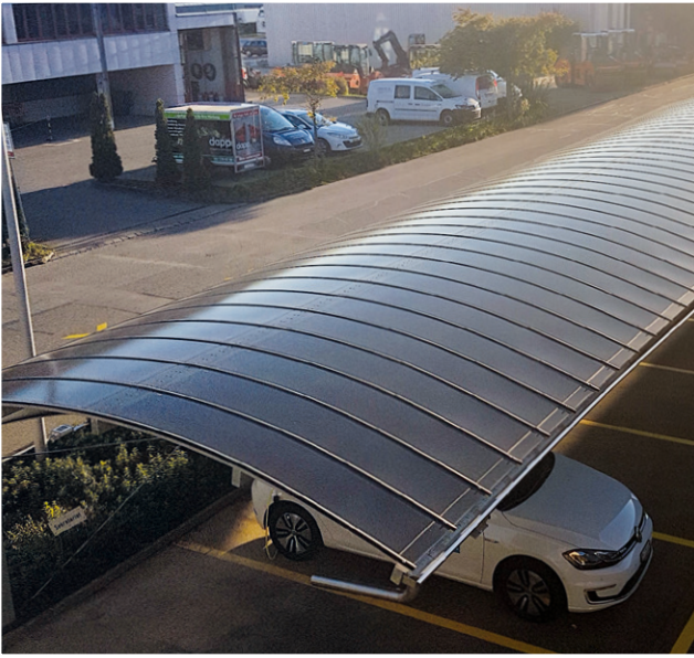
◀ Flexible CIGS modules can be curved over structures such as solar carports.
